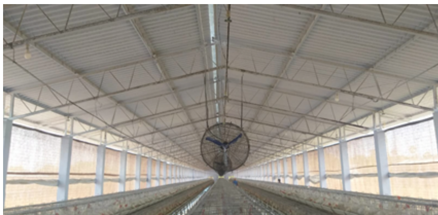
Fans increase air velocity within the house and create a cooling effect.
